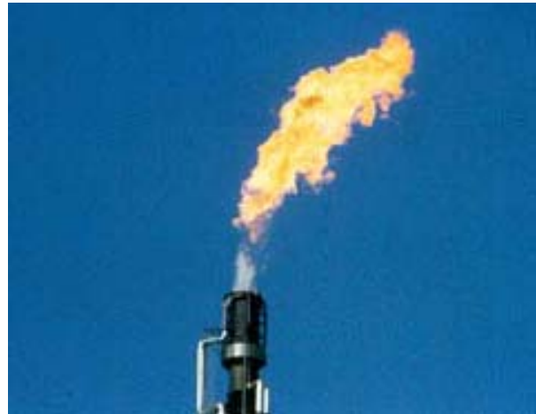
Figure 1. Flare stack Photo source: John Zink Company, LLC
