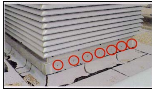
Adequate securement Source - FEMA
