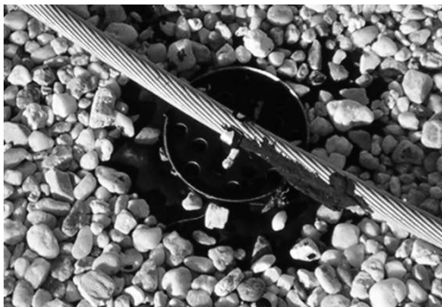
Conductor secured with clip adhered to cover
