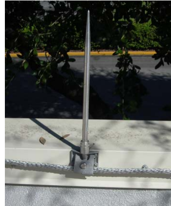
Air terminal screwed to wood nailer Source - FEMA
