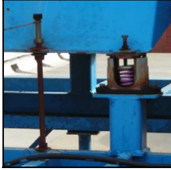
Vibration isolator with threaded rod for upward travel limit
