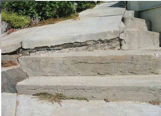
Photo 1: This stairway has high degree of variation in both riser heights and tread depths. If a riser is too high or too low, a person navigating the stairs may find it difficult to maintain safe footing. Treads that are too short force the stair user to either rest only part of a foot on each tread or to twist the foot unnaturally.
