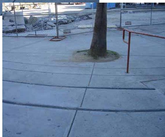
Photo 2: This half-round stair has an unusually long tread. The step edges could be made more conspicuous with hazard yellow striping and an intermediate handrail. Also note the deceptive visual cues created by nearby expansion joints, and the adjoining ramp handrail (to the right) which is excessively long.
