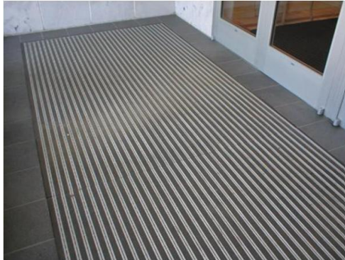
Vestibule with inlaid or recessed gridding *Courtesy of Lord & Taylor
