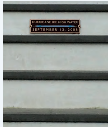
Hurricane Ike flood marks from September 2018. Source: Karen MacClune, ISET
